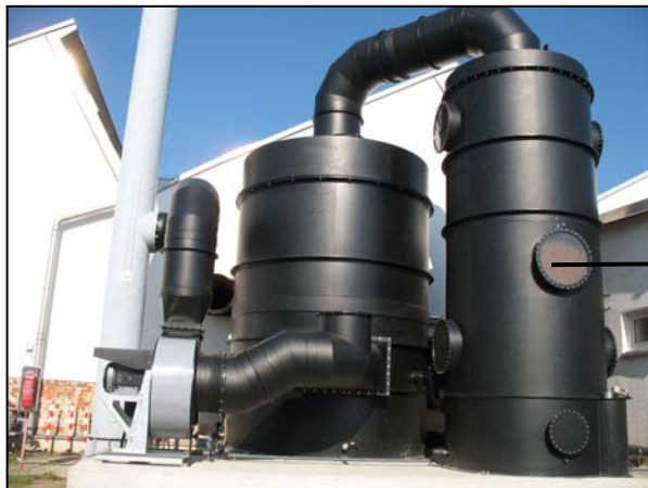
Filter-system for cleaning the waste gas in textile industry
